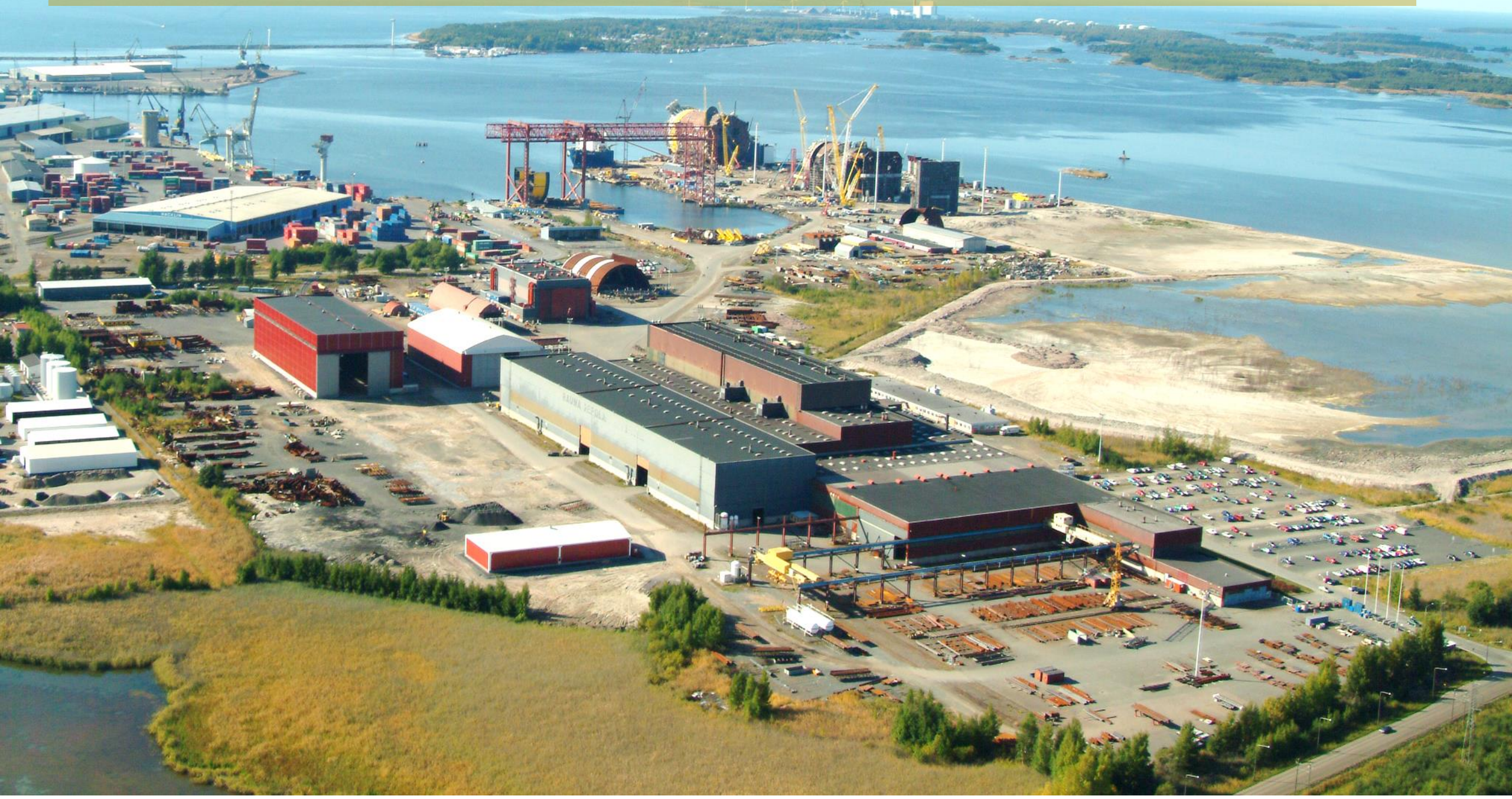
Floating wind foundation fabrication site: Hywind offshore energy project. Pori, Finland
